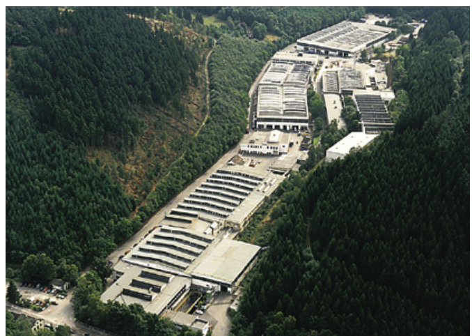
The Elspe plant seen from the air
